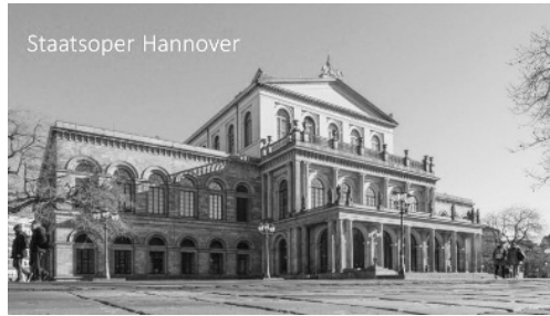
Fig. 4: Front view of the Hanover State Opera House. Photo: Clemens Heidrich, Hanover 2025
